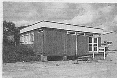
Fig. 2b The experimental building.
